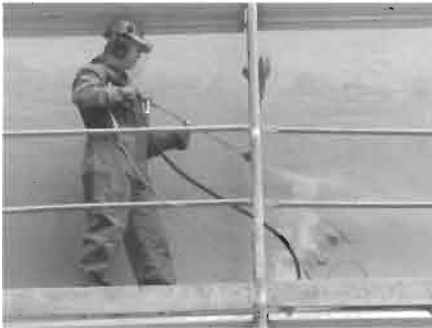
(c) Floor decontamination (Hammelmann GmbH, Oelde).
