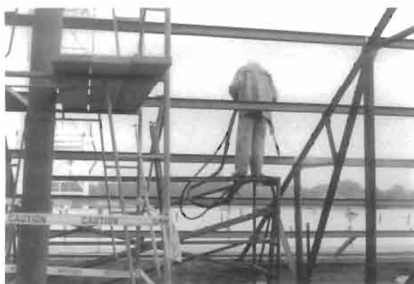
Figure 7.26 Use of ice jetting during a steel bridge rehabilitation project (photographs: Universal Ice Blast, Bellevue, WA).
