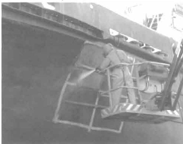
Figure 7.20 Ultra-high pressure abrasive blasting (UHPAB) systems in operation (photographs: Mühlhan Surface Protection Intl. GmbH, Hamburg).
