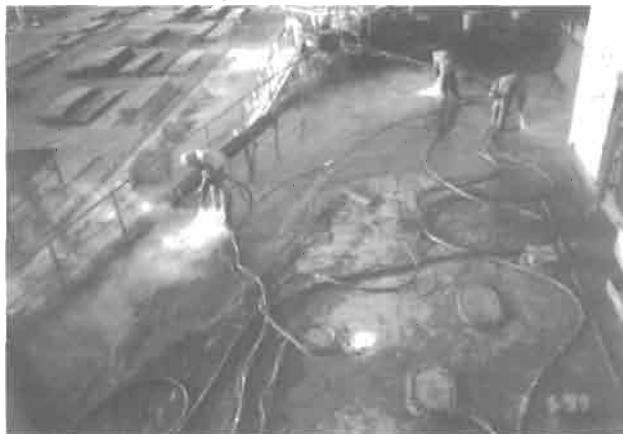
(b) Ship hull decoating.
